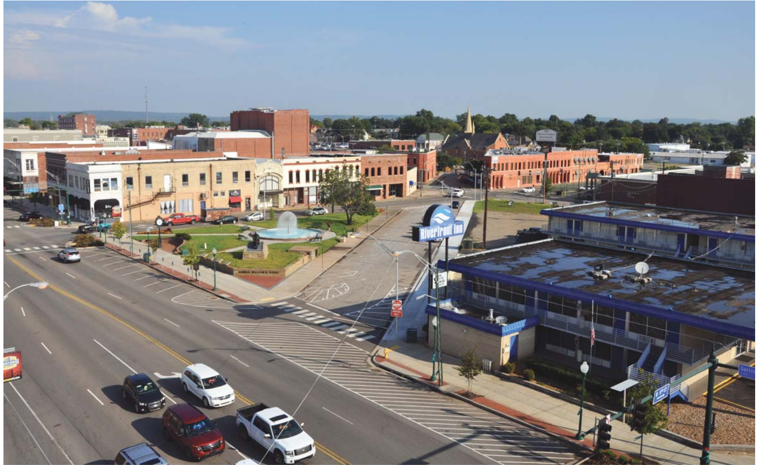
Existing Cisterna Park along Garrison Avenue and the Towson Avenue extension adjacent to the Riverfront Inn
