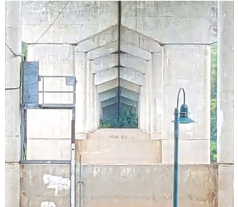
U.S. Highway 64 Bridge (Source: Gateway Planning)
